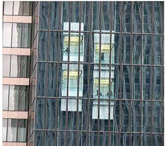
Figure 1: Double-deck Elevators at Midland Square, Nagoya, Japan (figure shown just to indicate the Double-deck design)
